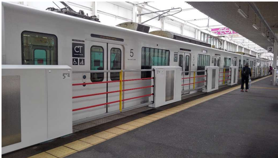
Lightweight platform door (JR Kyushu Kyudai Gakkentoshi Station)
