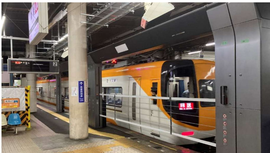
Elevating platform door (Kintetsu Tsuruhashi Station)
